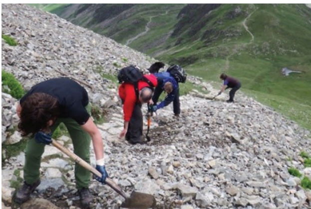
Repairing paths in the Lake District
